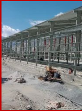
Pre Engineering Building Structure
