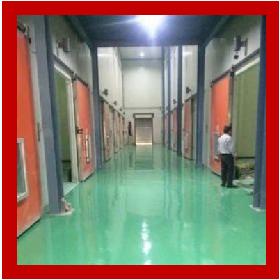
Controlled Atmosphere Cold Storage
