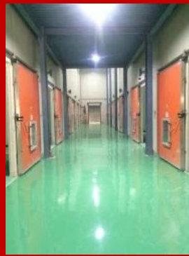
Controlled Atmosphere Cold Storage
